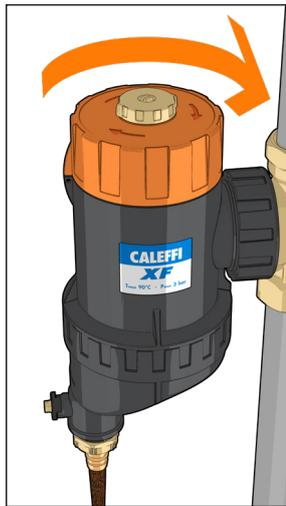
4. After cleaning, align the indicator on the top knob with the reference mark on the device body. Close the drain cock and start the system.
